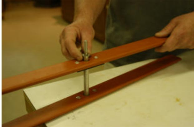
Turn the cedar post cap upside down and insert the threaded end of the bolt as shown.
